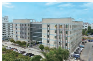
Building A2-1, Zedali Industrial Park, Zhancheng Community, Fuhai Street, Bao'an District, Shenzhen, China
